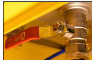
DRAIN VALVE IS CLOSED (HANDLE IN HORIZONTAL POSITION).
