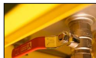
Drain Valve in Closed Position
