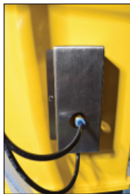
Cover in Place
