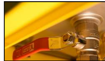
Drain Valve in Closed Position
